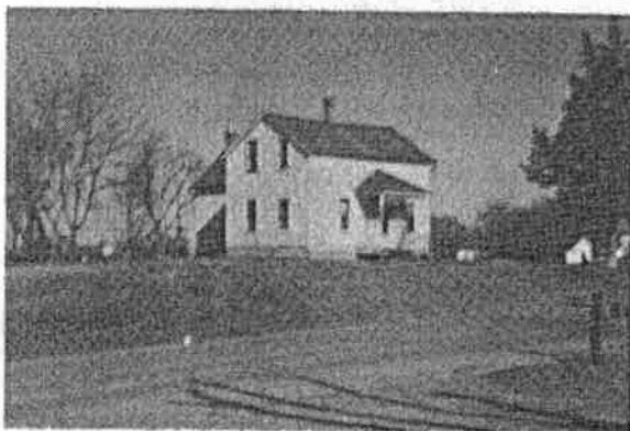
No. 2 is the home owned by Mr. & Mrs. John Heffern. John is a Lineman for the Municipal Utilities of New Prague. They live here with their family, with the exception of the two oldest who are living away from home.
